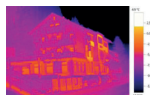
Thermal image with ScaleAssist
